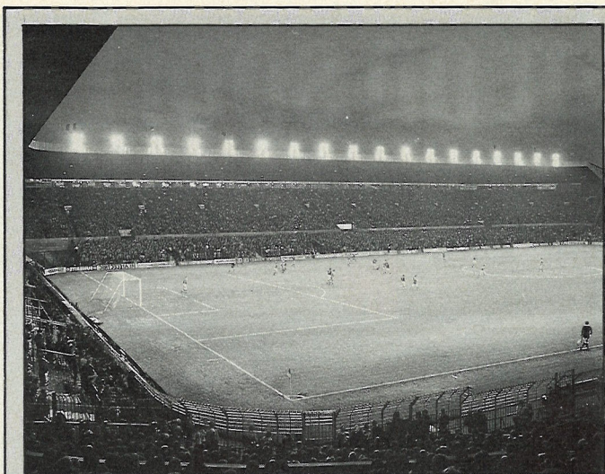
A new installation at Manchester United's Old Trafford football ground uses 216 asymmetrical Thorn OWA 1500 floodlights housing linear metal halide lamps to provide an average horizontal illuminance of almost 1500 lux. Floodlights are mounted in groups of six either side of the stadium. The installation replaces an earlier scheme based on four corner towers which provided an average illuminance of only 800 lux.
